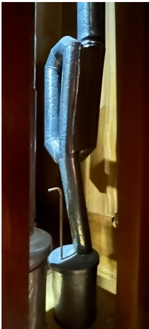
A pipe which has been bent (mitered) to fit in a small space, but which cannot support its own weight.
